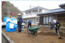
● Scraping off of garden soil, etc. (Provided by Date City)
