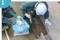
● Cleaning of eaves and gutters of private houses
