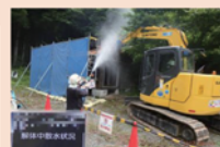
Demolition of a damaged house, etc.
