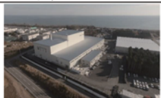
Temporary Incineration Facility in Okuma Town (December 2017)
