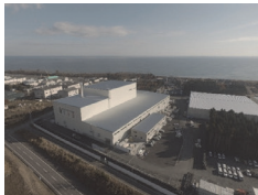
Temporary Incineration Facility in Okuma Town (December 2017)
