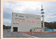
Temporary Incineration Facility in Naraha Town (Oct. 2016)
