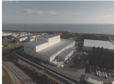
Temporary Incineration Facility in Okuma Town (December 2017)
