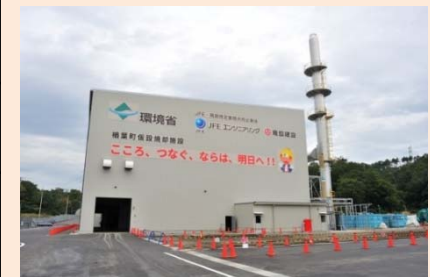
Temporary Incineration Facility in Naraha Town (Oct. 2016)
