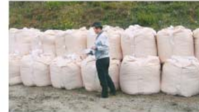
Flexible containers (filled with removed soil)
