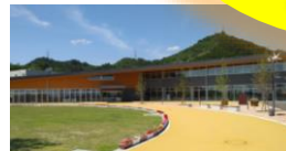
Introduction of a solar power generation system to the Okuma Town Office Building
