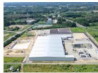
Non-combustibles recycling facility
