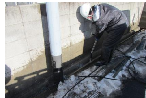
● Removal of sludge from ditches (Provided by Fukushima City)
