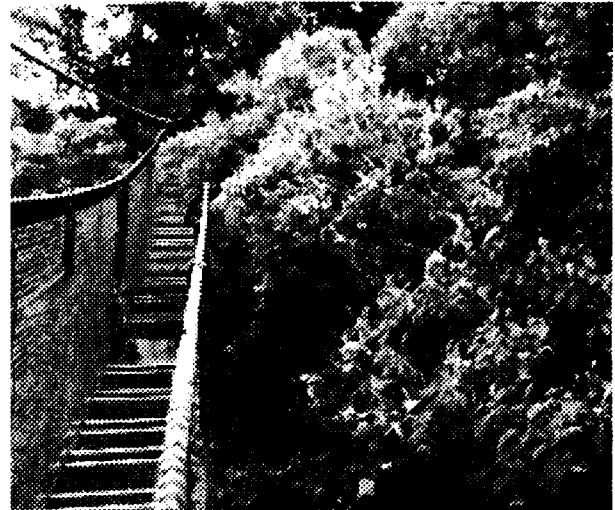
Fig. 4 The horizontal moving section set on the canopy
