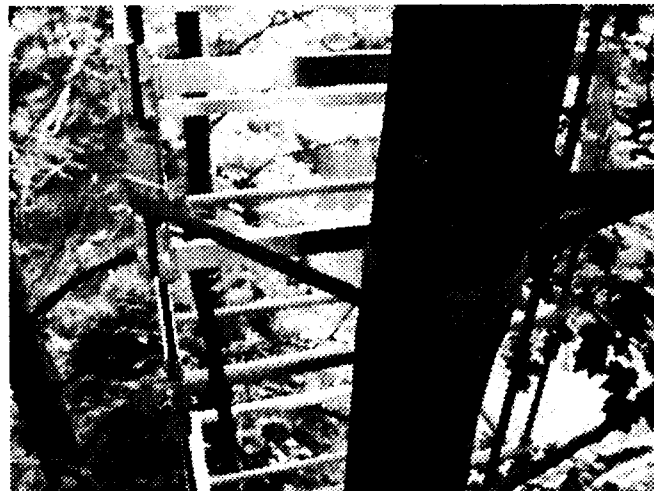
Fig. 7 Slings the connecting frame to the stem
