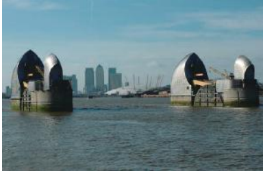
On the river mouth, the Thames Barrier is designed to protect inland areas from storm surges until 2030, even if sea level rises 8 mm per year.
