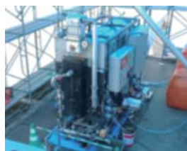
Trial Running at Treatment Plant
