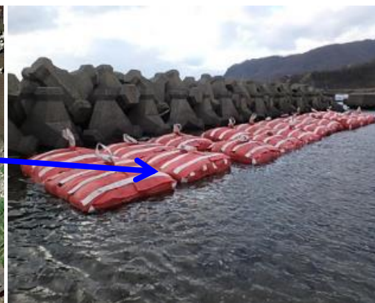
Installing Vivary™ Rocks as a substrate material for seaweed settlement
