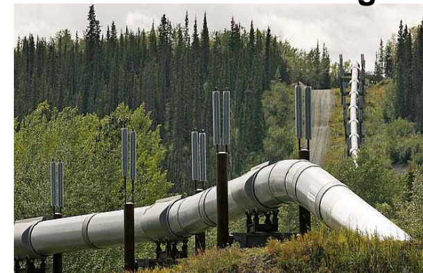
Reducing pipeline leakage
