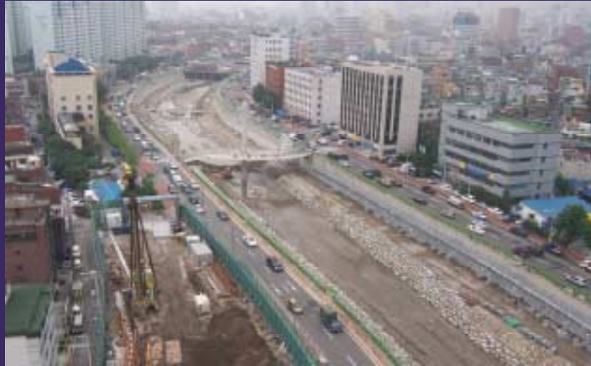
The view of downstream(Sector 3) the progress of construction : 76.70 %
