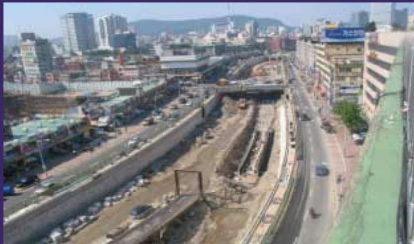
The view of mid-stream(Sector 2) the progress of construction : 74.98%
