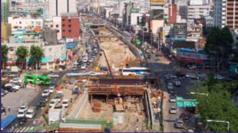
The view of upper stream(Sector 1) the progress of construction : 70.80%
