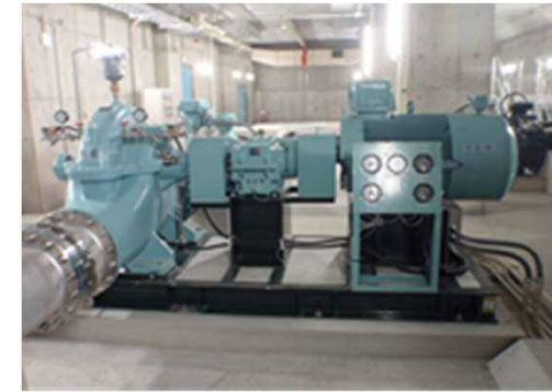
Hydroelectric power facility
