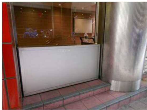
Flood stop doors
