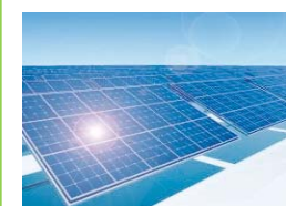
PV Power Generation (Roof-Top) in Bus Port 51KW
