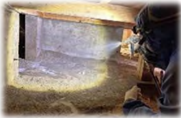
Chemical application under the floor
