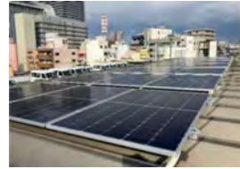
Multi-story Parking Facility for Official Vehicles (Solar power systems & battery storage)
