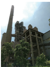
Hai Phong Cement
