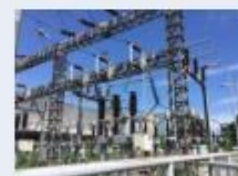
High Efficient Transformer
