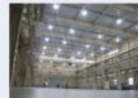
Indoor LED Lighting
