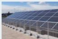
PV system with batteries
