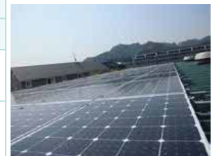
Solar power generation system
