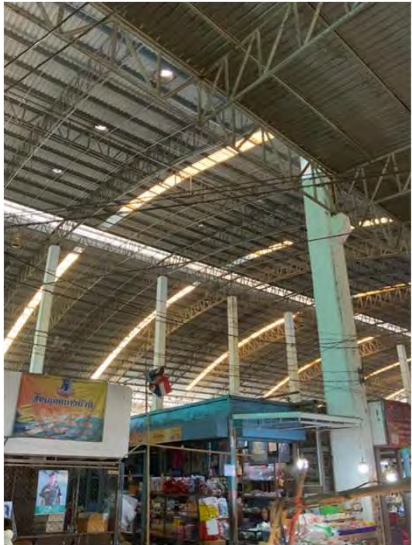
Roof at the Market
