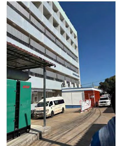
Concrete Building (area for solar panel installation)
