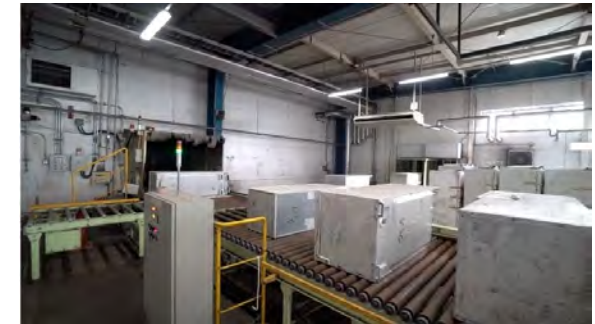
To the crusher
