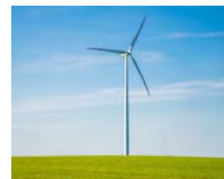
Solar power, wind power, other
