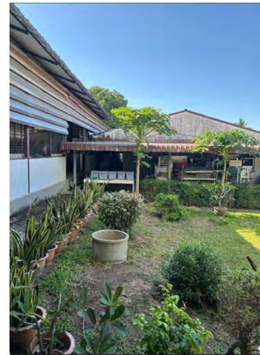
Roof of Temporary Building
