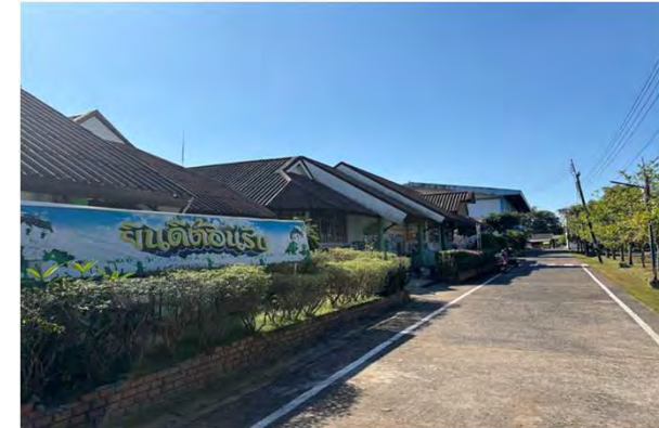
Appearance of Roof (Kindergarten)
