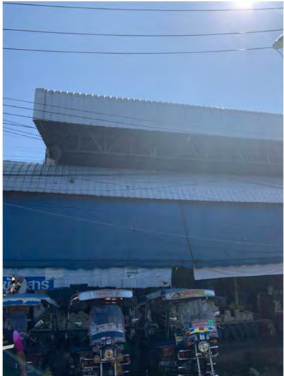
Appearance of the Roof
