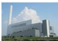
Waste to Energy Plant
