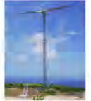
Retractable wind turbines in Awaguni-Island
