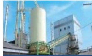
Biomass Co-Generation System, Fuji-Foods Corporation, Thailand
