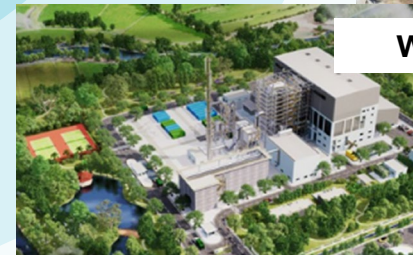
Waste to Energy
