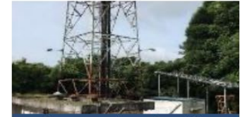
Energy-saving of mobile communications base transceiver stations, KDDI Corp. Indonesia
