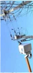
• Incoming Line Construction
