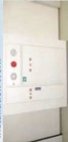
• Indoor Fire Hydrant Installation Work
