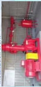
• Powered Fire Pump Installation Work
