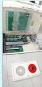
• Fire Alarm System Installation Work
