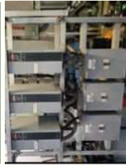
Installation of Variable Frequency Drives
