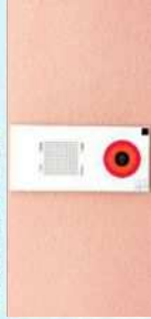
• Emergency Alarm System Installation Work
