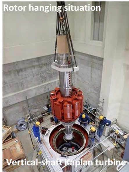
Vertical-shaft Kaplan turbine
