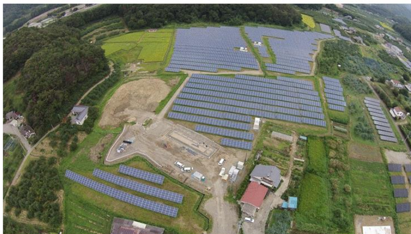
Large-scale solar power generation facility within city limits (photo by Apollo Gas Co., Ltd.)
