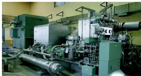
Steam turbine generator
