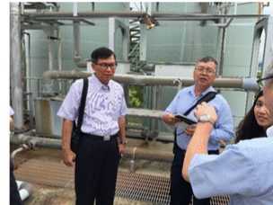
Biogasification of Effluent at a Food Factory (Methanation→Gasification generation)
