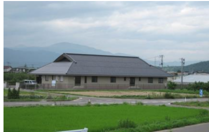
Drainage treatment plant in Yamaguchi District
