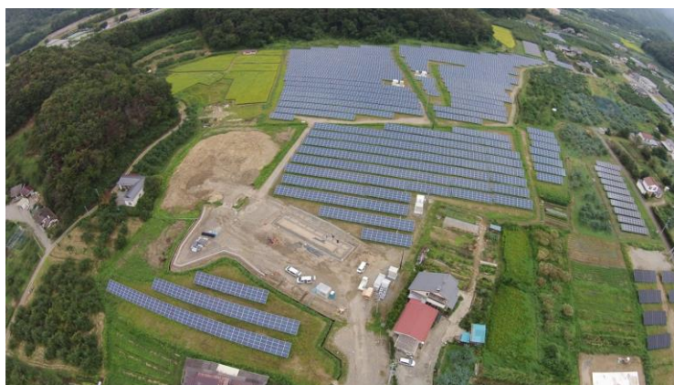
Large-scale solar power generation facility in Fukushima City (Photograph provided by Apollo Gas Co., Ltd.)
