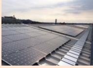
Solar power generation facilities
