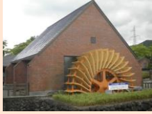
The Village of Four Seasons' small hydro power generation facility leverages local resources and the technologies of a local corporations .
