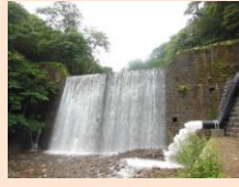
Small hydro power plant utilizes check dams
