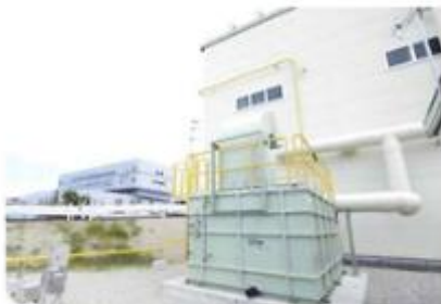
*Active carbon filter deodorization equipment (left) *Photocatalytic deodorization equipment is installed on the roof of the sludge receiving building (right)
