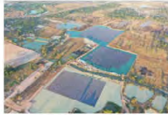
Floating Solar PV, TSB Co., Ltd., Thailand
