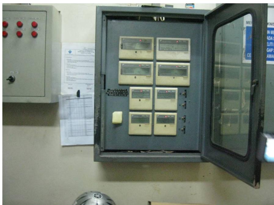
図 5.2-8 Central remote controller and Schedule timer in Basement floor control room
