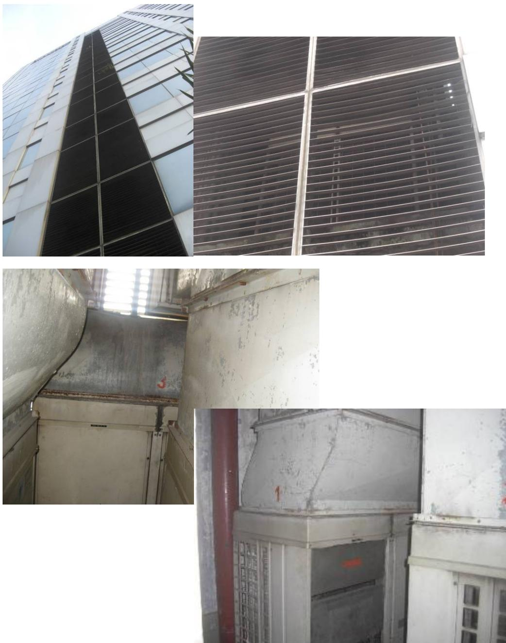
図 5.2-4 Outdoor unit for 7<sup>th</sup>-16<sup>th</sup> Floor located in each floor Mechanical room
