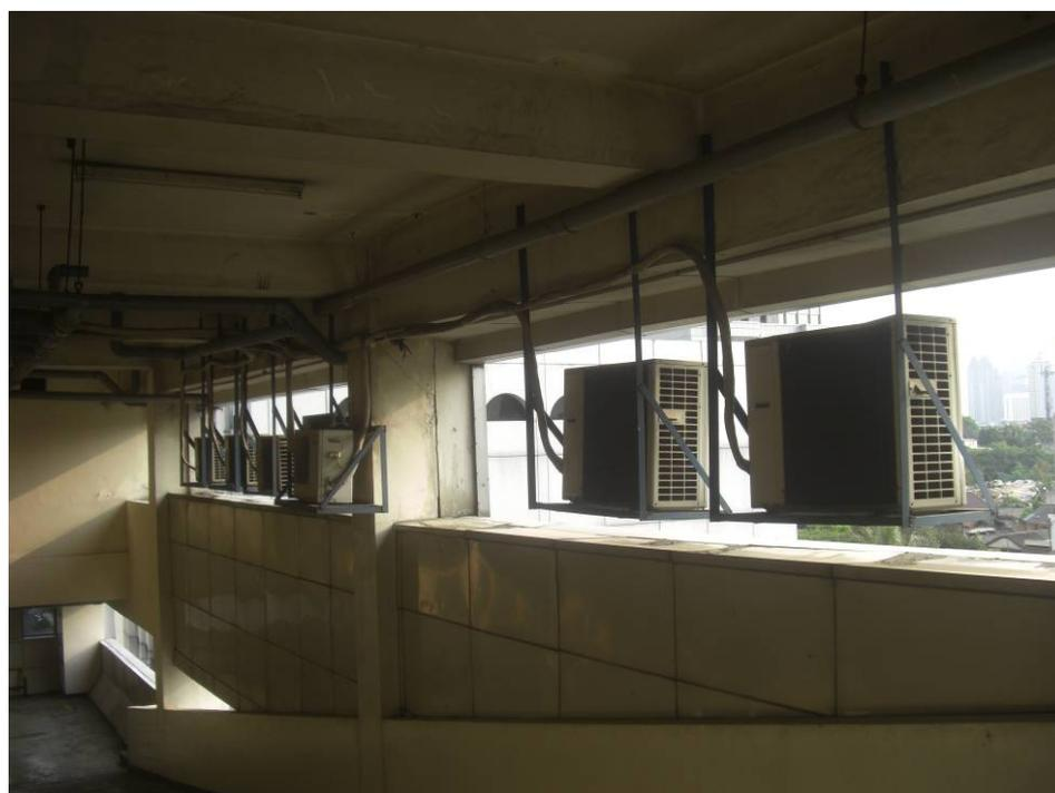
図 5.2-7 Many separate A/C are added on roof and parking
