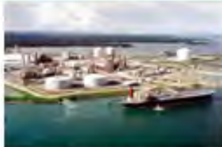
Methanol plant (East Kalimantan Island, Bontang)
