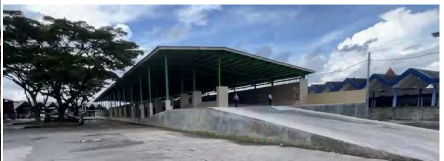
Waste treatment plant "RA-X"
