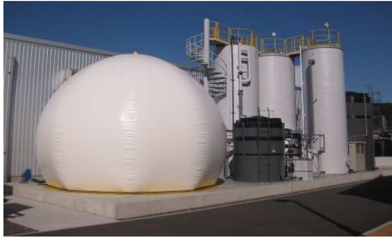
UASB methane fermentation for liquid waste UASB : Upflow Anaerobic Sludge Blanket
