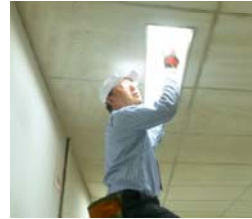
Installation of CCFL
