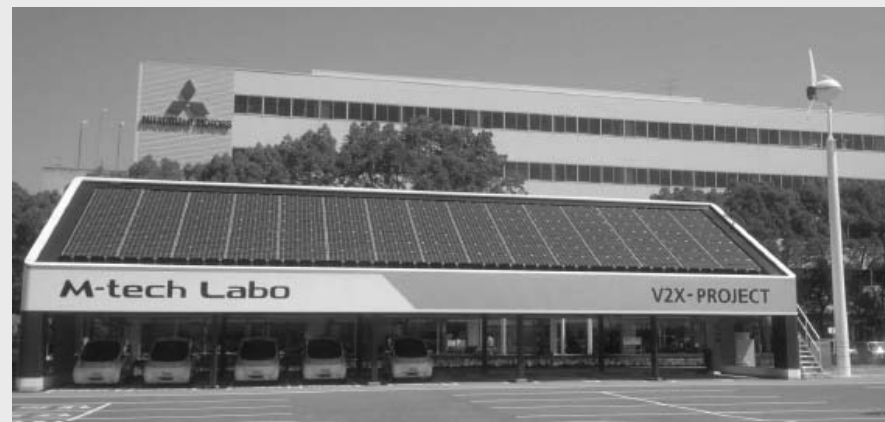
To supply power to factory
