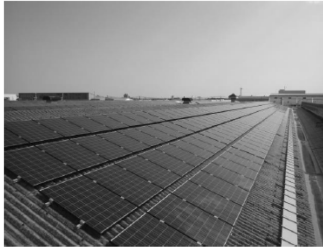
Factory roof after installation
