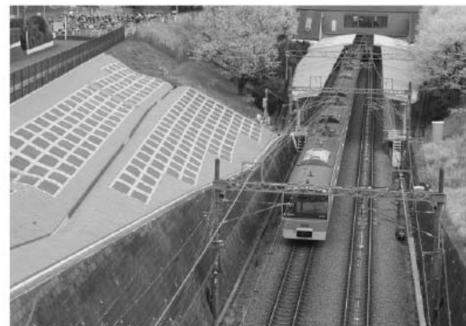
Railway slope after installation
