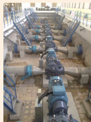
Installed high-efficiency pumps
