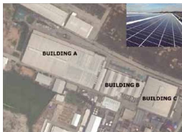
Figure 29. PV power generation facility on the roof of a factory (©Fine Tech Co., Ltd.)
