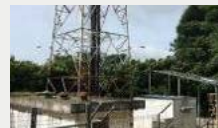
Energy-saving of mobile communications base transceiver stations, KDDI Corp. [Indonesia]
