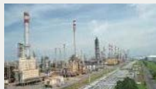
Optimization in petroleum refining plant, Yokogawa Electric Corp. [Indonesia]
