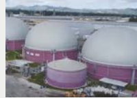
Biogas Power Generation, ITOCHU Corporation, [Philippines]
