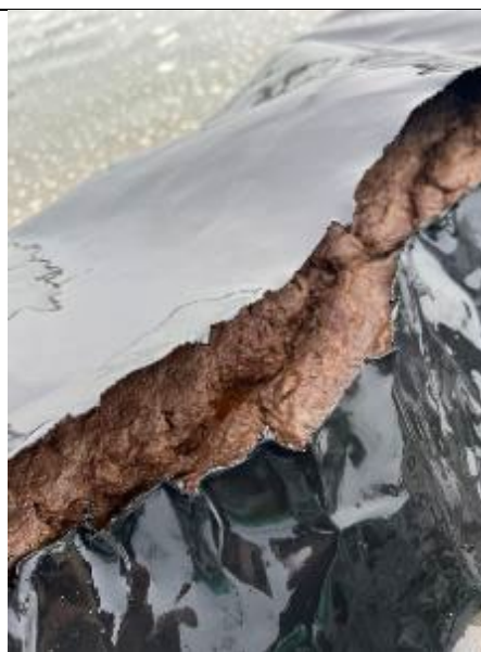
Plastic sheet is placed to cover the bottom of the aquaculture pond
