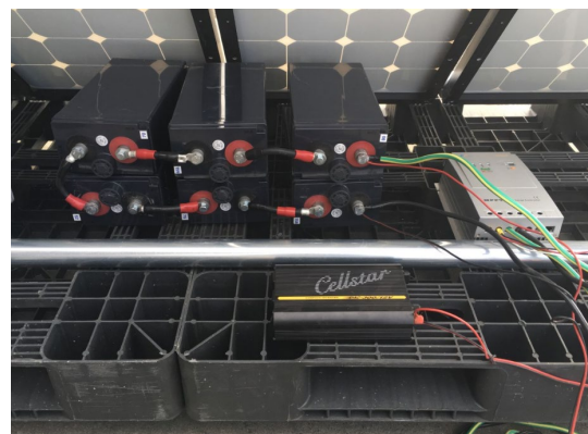
Figure 2.1.1.2. Small-scale, stand-alone power supply unit (Source: IGUAZU Corporation)
