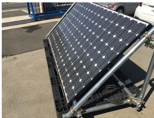
Figure 2.1.1.2. Small-scale, stand-alone power supply unit (Source: IGUAZU Corporation)
