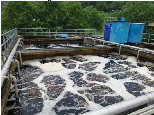
Leachate treatment facilities (aeration tanks)
