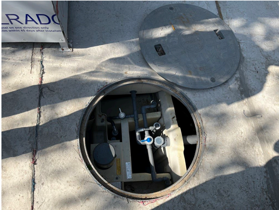
Photo 13: Johkaso in almost complete condition (November 25, 2023)
