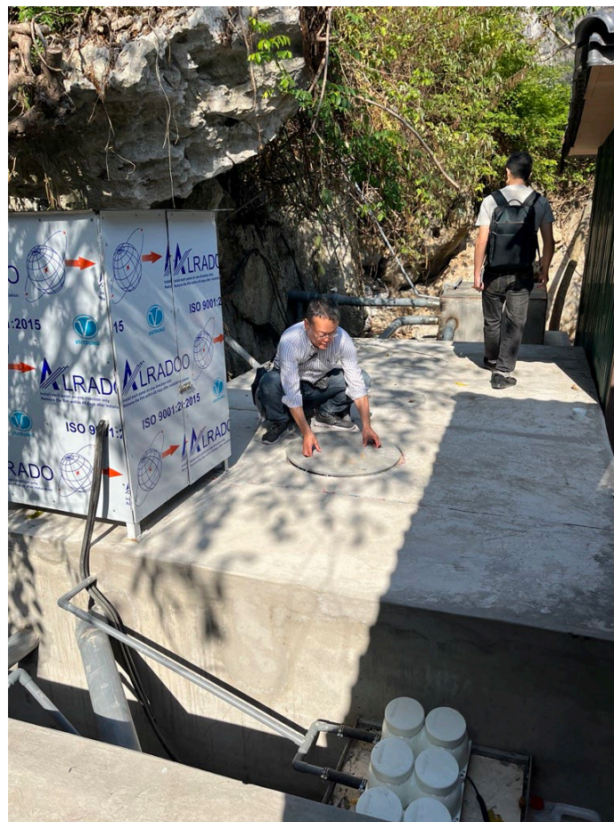
Photo 12: Johkaso in almost complete condition (November 25, 2023)
