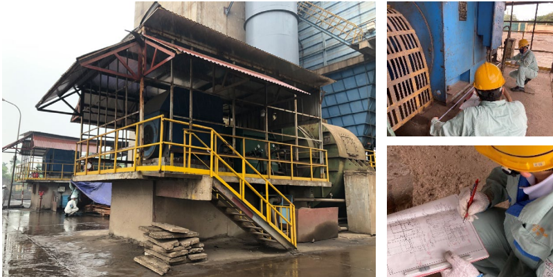
A large industrial blower that is scheduled to be applied for the JCM Model Project and a site survey
