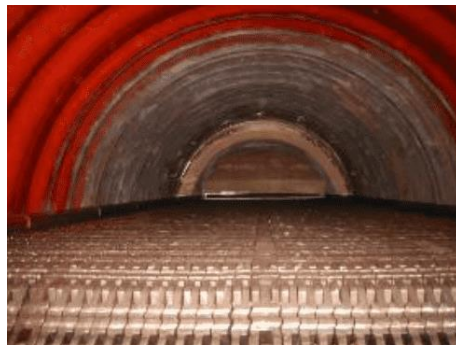
Figure79 Inside the Stalker (Chain Grate)
