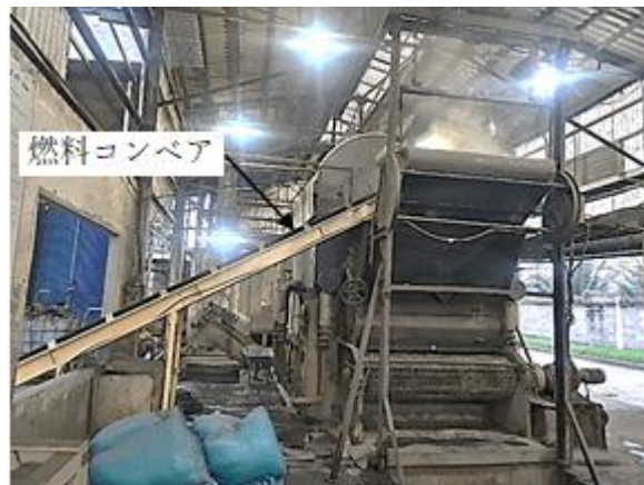
Figure75 Vietnam made natural circulation boiler (moving floor stoker-fired) at CJ Agri
