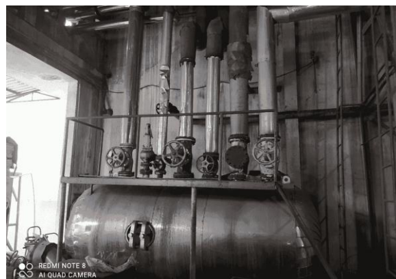
Figure60 Thermal oil boiler
