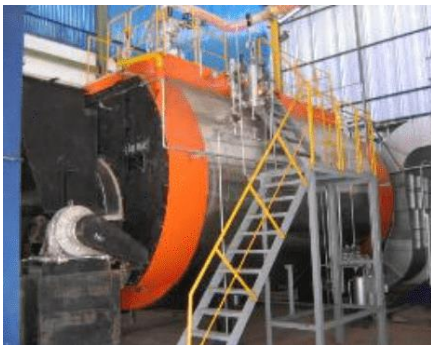
Figure80 Cylindrical boiler
