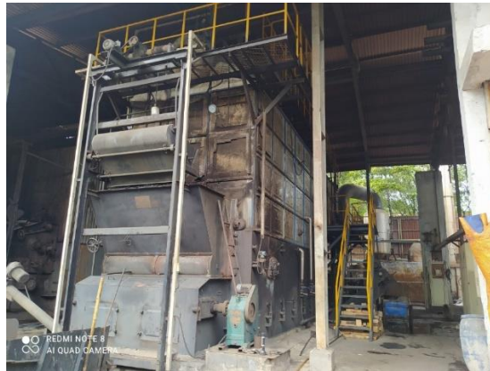
Figure66 Vietnam made single-body natural circulation boiler (moving floor stoker-fired), AGTEX28
