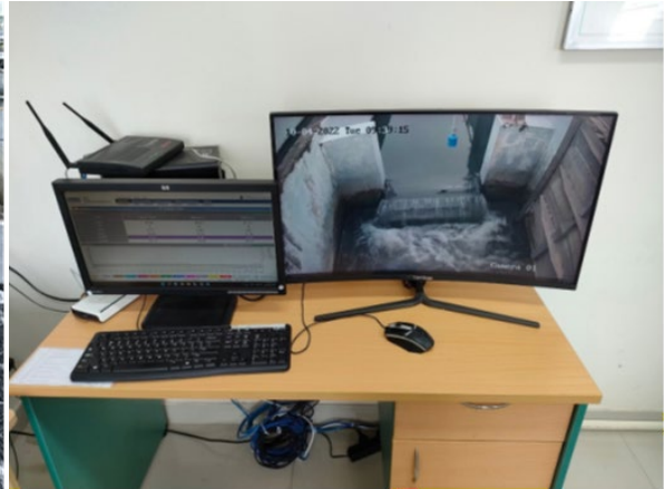
Monitoring of the wastewater treatment facility
