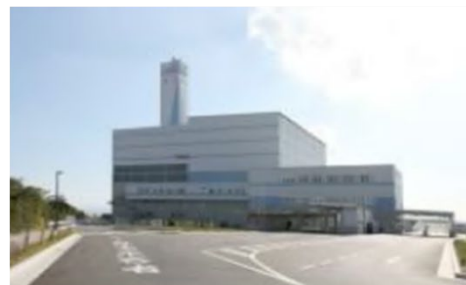
Clean Center Waterfront Plant (Melting treatment* and waste to energy) * Solid waste is melted at high temperatures of 1,700 to 1,800 Degrees Celsius. Metallic waste is recycled as metal, and other waste is recycled as slag.
