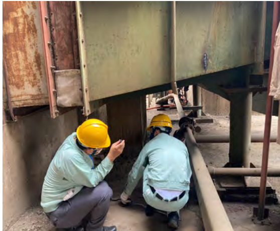
Field survey (checking existing blower duct section)
