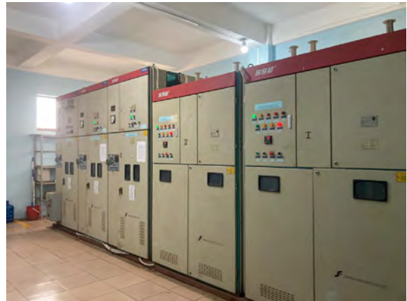
Field survey (checking electrical room)
