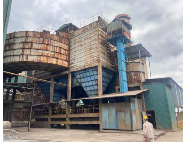
Equipment covered by this survey (rear exterior view)
