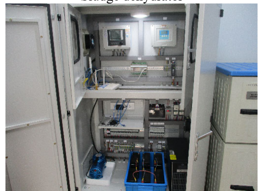
Wastewater monitoring system
