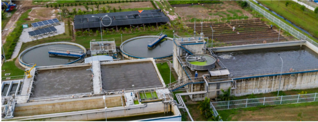
Aerial view of wastewater treatment facility
