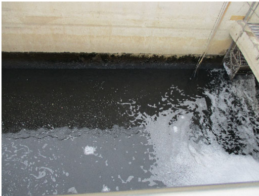
Water receiving tank
