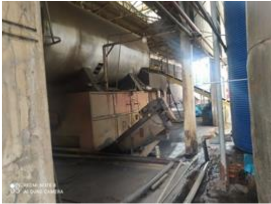
Figure 57 Slag Discharge System at the bottom of furnace (right), Conveyor to feed Rice Husk Pellet (left)
