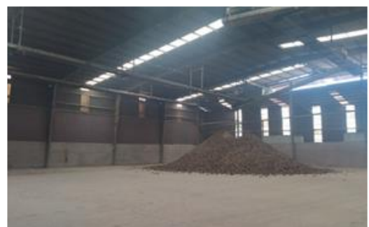
Figure 34 Space available for installation of Grind Mill
