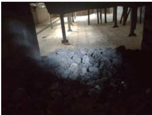
Figure 41 Coal inlet to the combustion furnace (Combustion gases enter the lower part of the drying chamber.)
