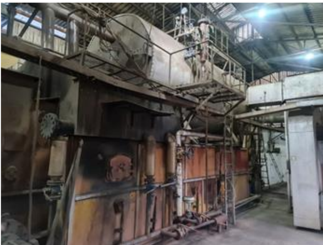
Figure 56 Combustion chamber and the section of water tube boiler
