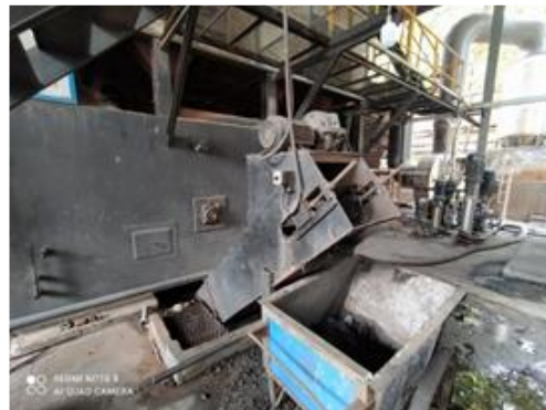
Figure 52 Discharge system for furnace bottom slag
