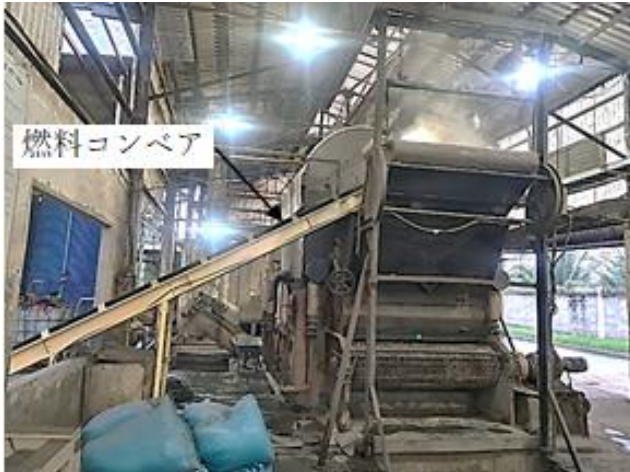
Figure 55 Vietnam made natural circulation boiler (moving floor stoker-fired) at CJ Agri Vietnam
