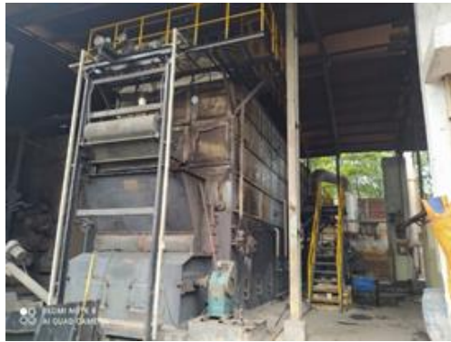
Figure 48 Vietnam made single-body natural circulation boiler (moving floor stoker-fired), AGTEX28
