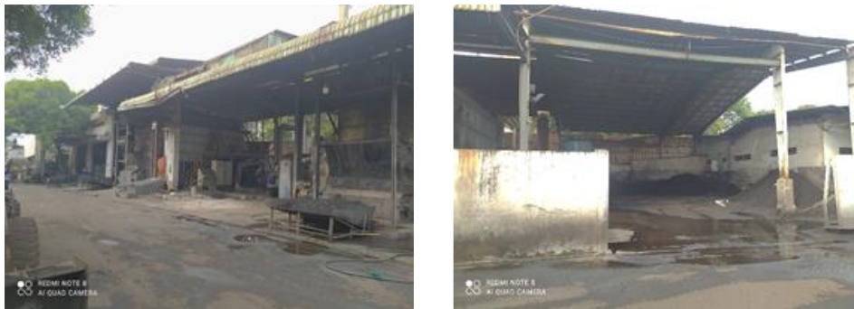
Figure 49 Boiler and coal storage area
