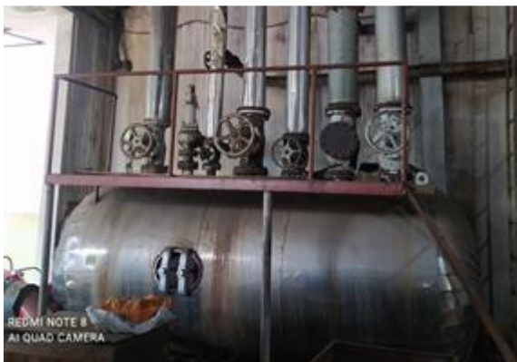
Figure 45 Thermal Oil Boiler
