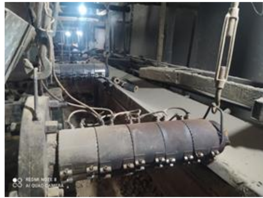
Figure 32 Conveyor belt that feeds briquette
